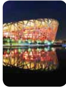
CHINA Beijing National Stadium
