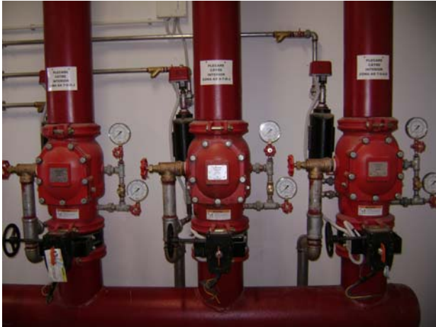
Victaulic FireLock NXT™ Series 751 wet devices
