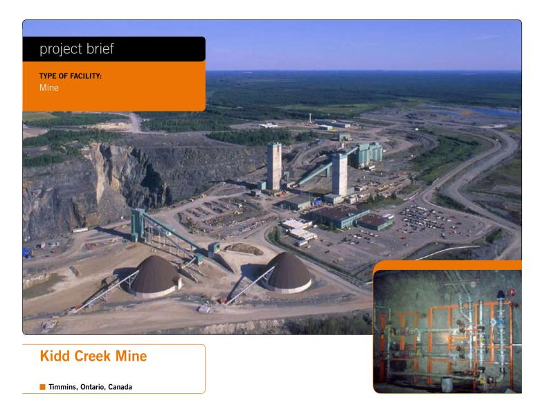
Kidd Creek Mine is a leading producer of copper, zinc, and other base metals since 1966. With a current depth of 9,100ft/2,774m a solution was required to ensure underground process water is distributed throughout the mine at reasonable working pressures.
