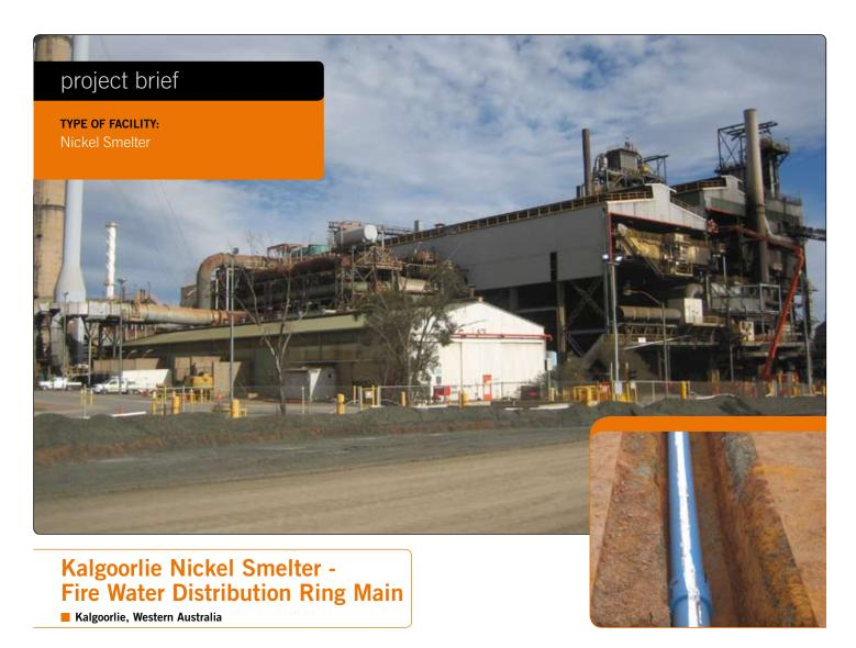
As part of the Kalgoorlie Nickel Smelter upgrade a new fire water ring main was installed around the site with a large majority of the pipes being buried service applications.
