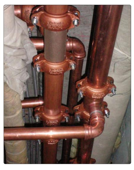
The Arbour Glen Condominium on 212 Kerr Street in Oakville is a 10-story, 100 unit building built in 1974. Needing replacement of all hot and cold domestic water lines, a flame free solution was desired so tenants would not be inconvenienced.
