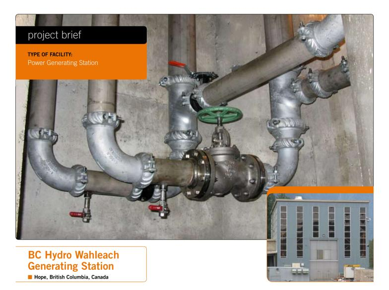
The BC Hydro generating station at Wahleach Dam was constructed in 1952 and produces 60 MW of power. When a new piping system was required for turbine cooling water, BC Hydro enforced a fast-track schedule in efforts to minimize downtime which could cost thousands of dollars per day.
