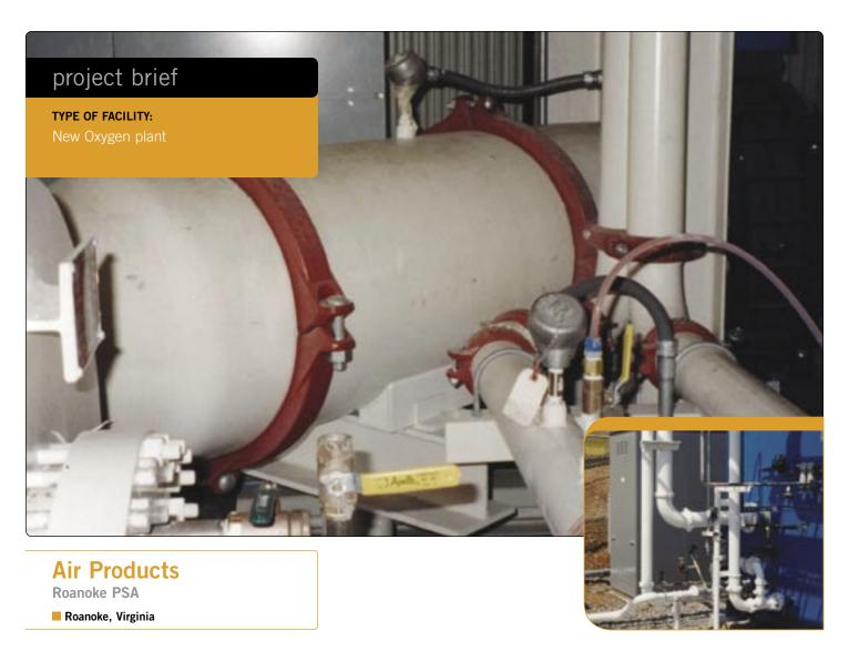
When Air Products built a new oxygen production plant in Roanoke, Virginia, Victaulic grooved piping products were used on oxygen and nitrogen lines, for their ease of maintenance.
