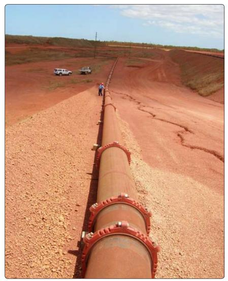
The project required the construction of an 8KM tailings line around a large tailings dam which had an oval plan shape. The dam shape necessitated deflection at the pipe joints for the pipe line to remain in the required position on the dam wall.
