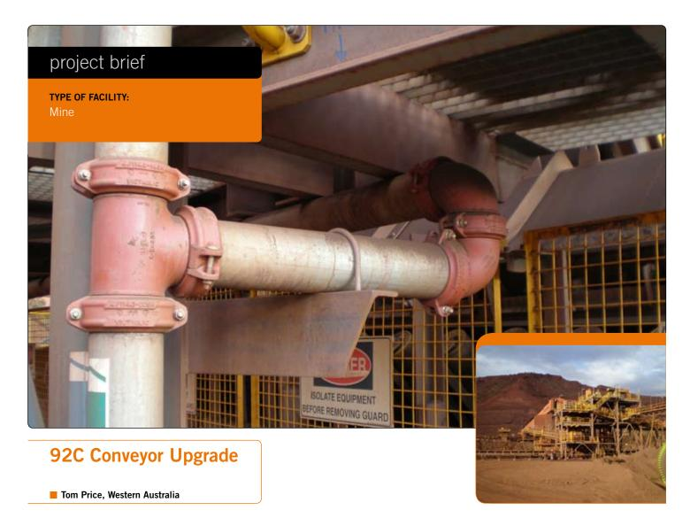
Pilbara Iron recently installed new conveyor belts at the Tom Price Iron Ore Mine, where Victaulic was utilised along the whole length of the conveyors for fire protection services.
